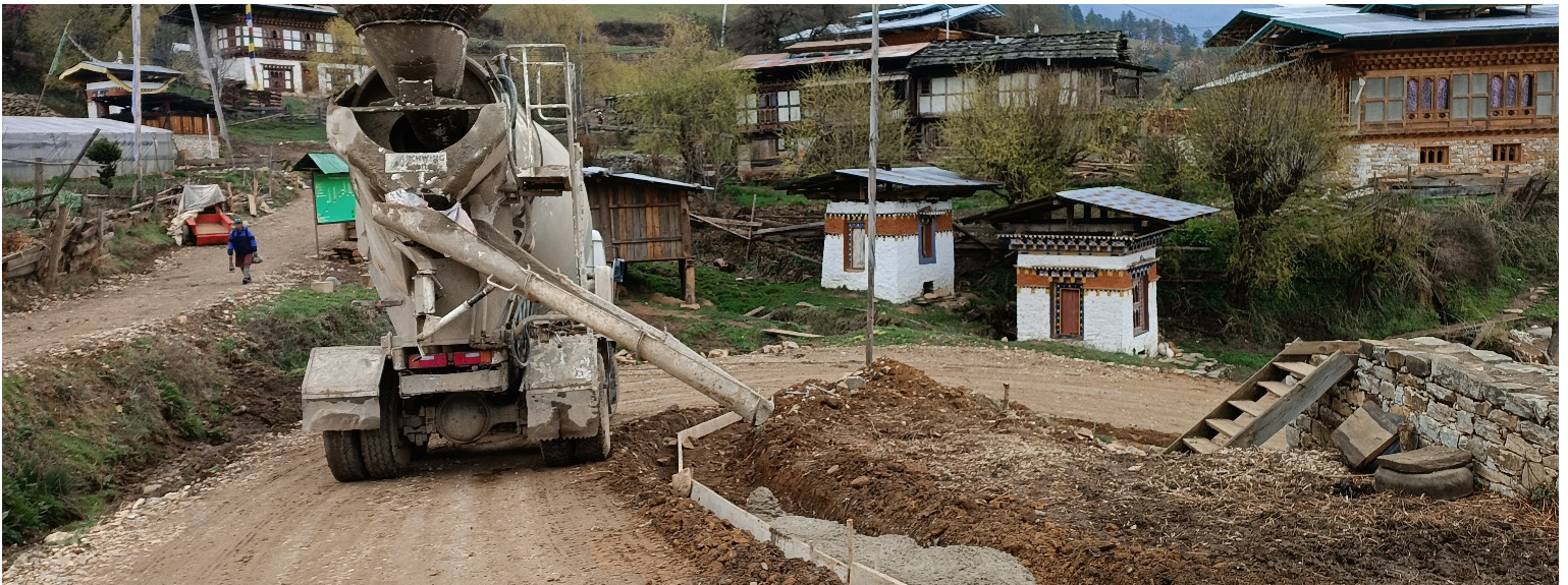
Work on the drainage of the road
