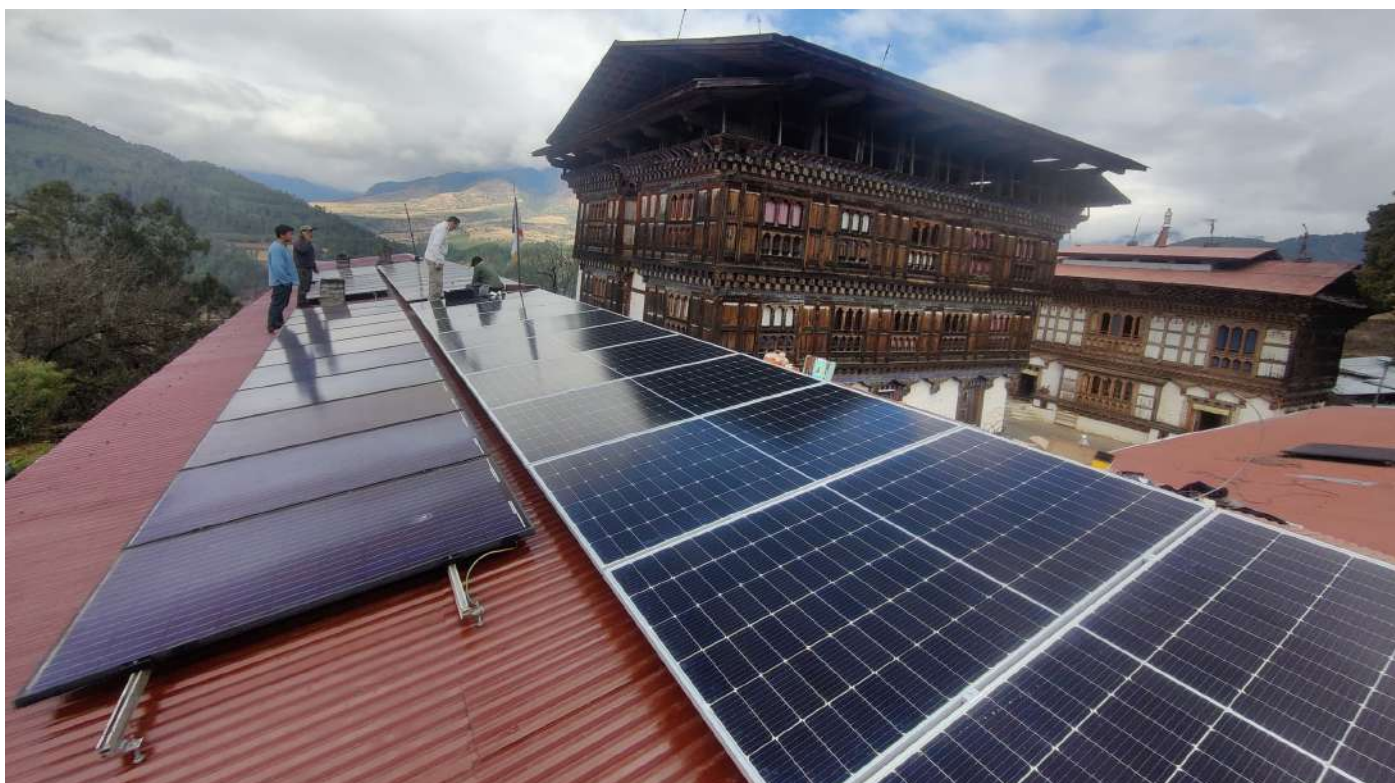
Installation of the solar panels
