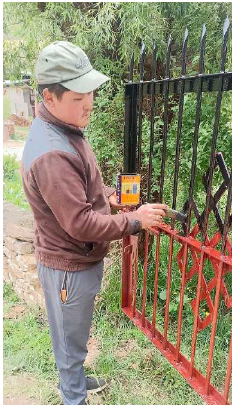
Chador Tshering painting the newly installed gate
