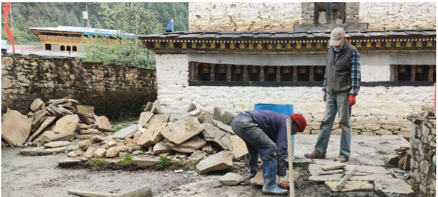
Master Mason Ap Phola laying out the stone slabs
