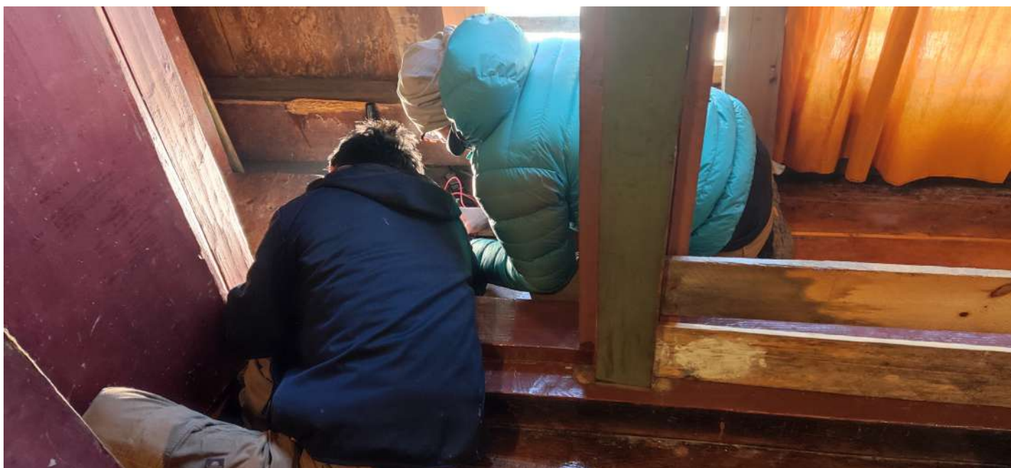
Eduard Wirth and Dorji replacing wires for the alarm system
