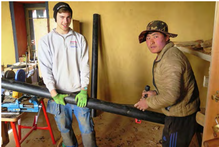
Nico and his assistant Chador welding pipes
