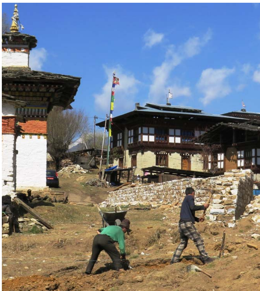
Masons working on the boundary wall
