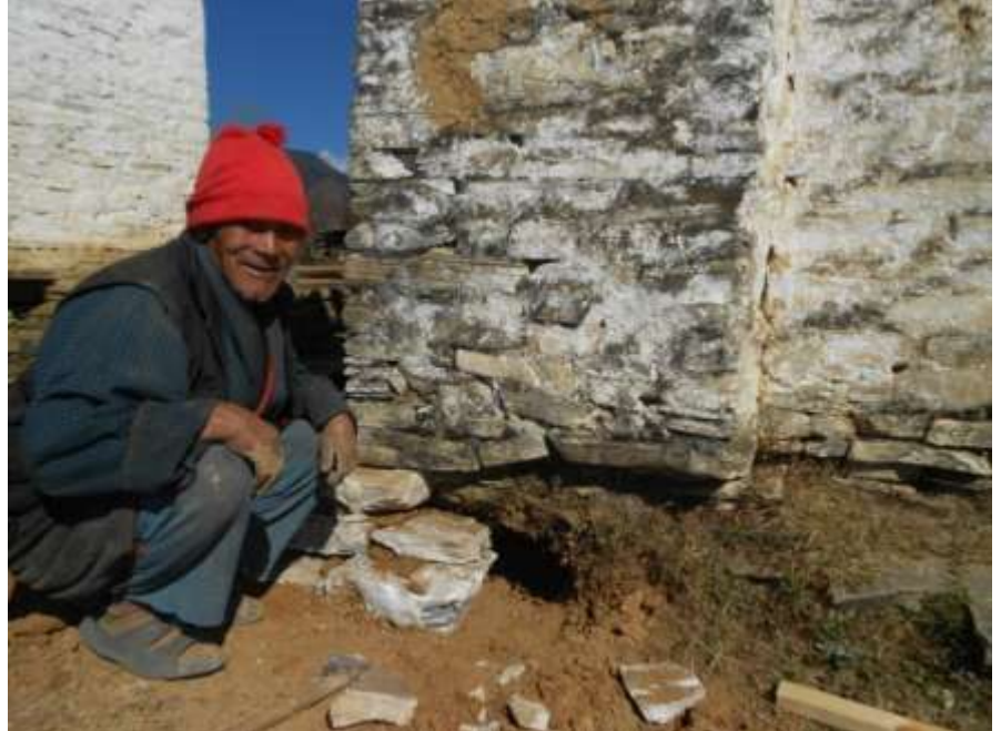
Picture: The completely reworked entrance steps and gate
