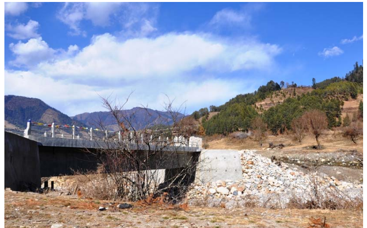
New bridge over Tang river
