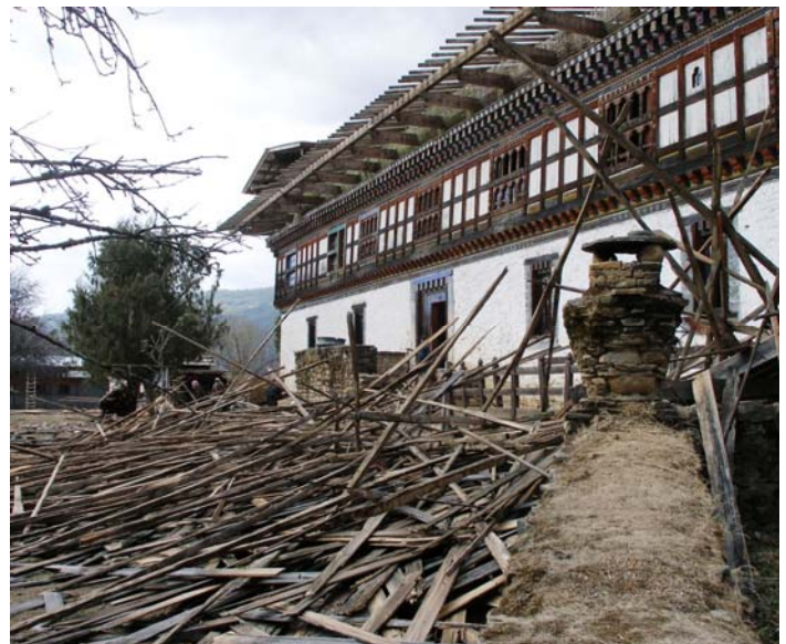
Roofing of shakor under progress (east side)
