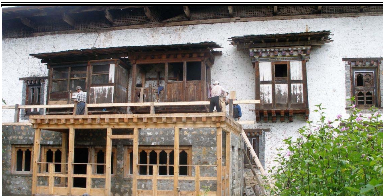
Kitchen and bathroom annex (west side)
